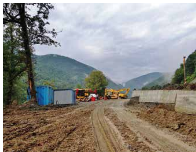
Fig. 4. Development of new roads into the Western Caucasus World Heritage property.
