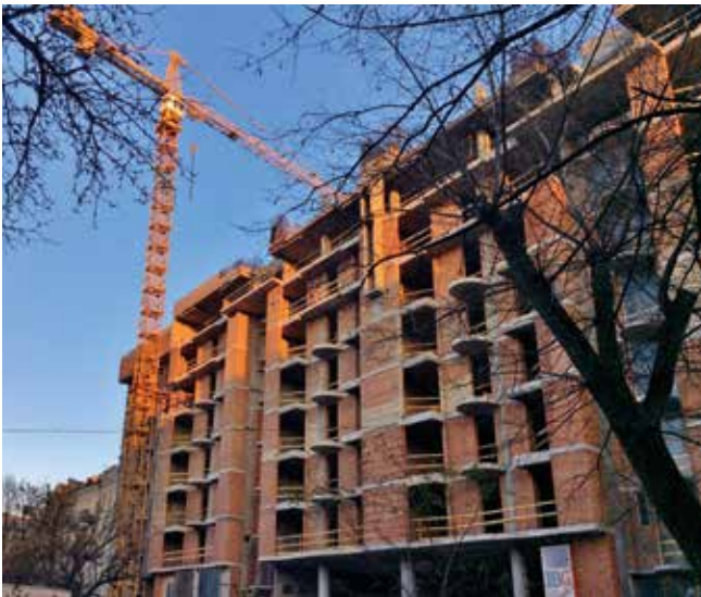
Fig. 2: The new construction at Gonchara str., 17-23.
