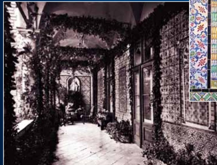
View of the 1st-floor loggia, 19th c.
